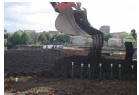
TERRAM Geozellen, 250mm x 150mm, 7m x 5m Abmessung
